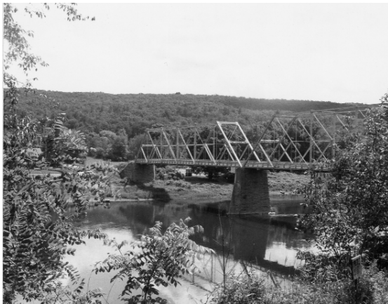
Skinnners Falls Bridge 1902
