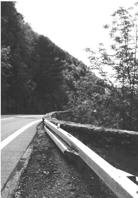
The insensitive placement of this guide rail diminishes the integrity of the stone wall at Hawk's Nest. Relocation of guide rail recommended.
