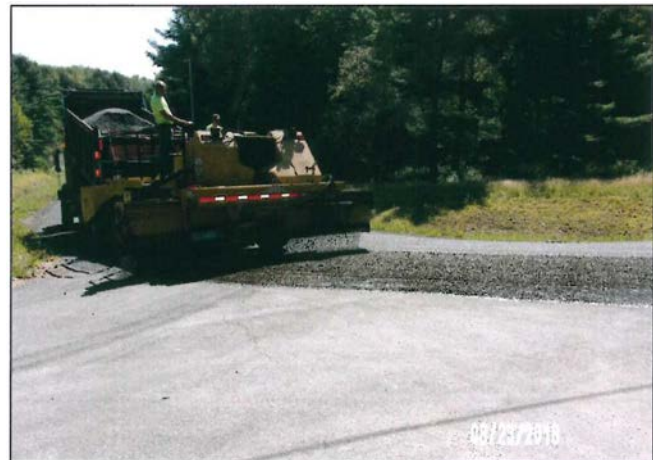
CR 74-Chip Sealing (Oil and Stone)
