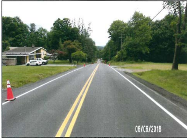
CR 109-Road Striping
