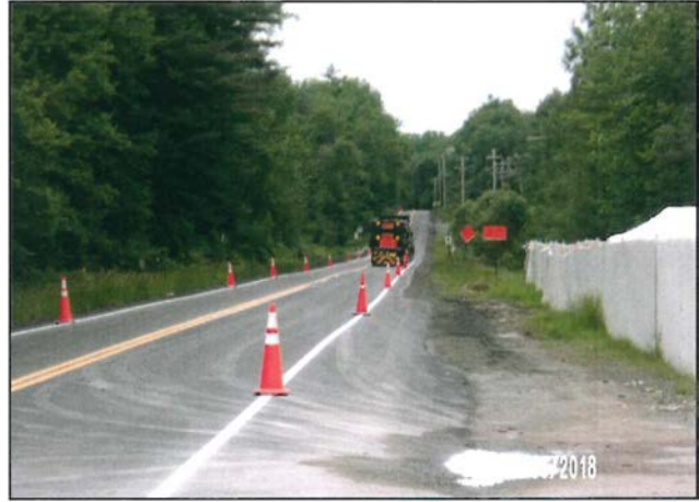
CR 59-Road Striping
