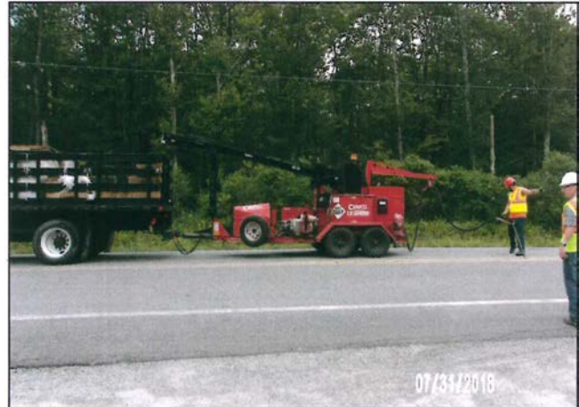
CR 96-Crack Sealing prior to Chip Seal
