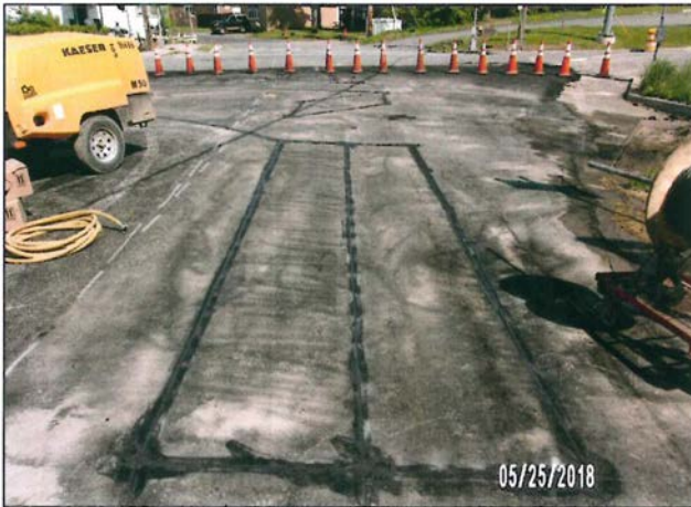
CR 109-Traffic Light Loop Installation
