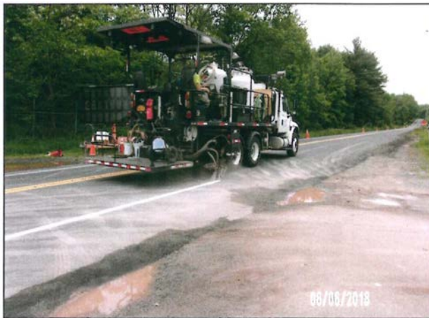
CR 59-Road Striping
