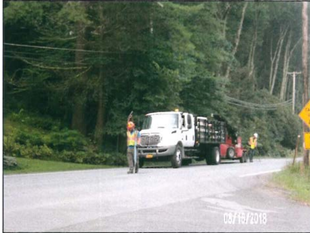
CR 19-Crack Sealing prior to Chip Sealing
