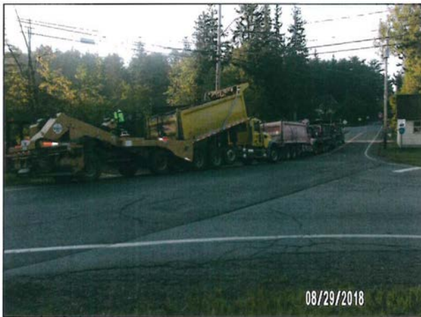
CR42-Chip Sealing (Oil and Stone)
