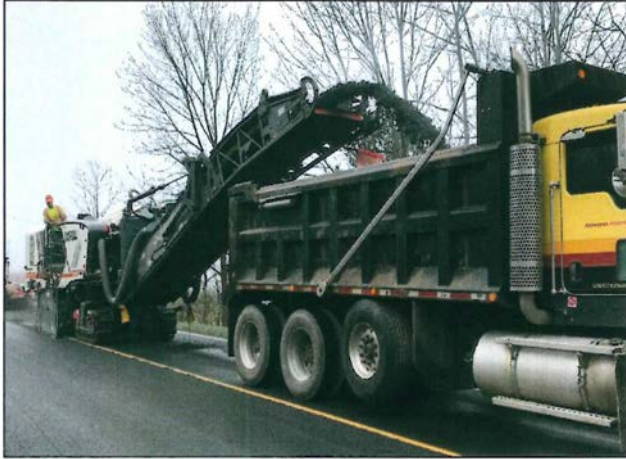
CR 143-Milling for Partial Depth Repair Sections
