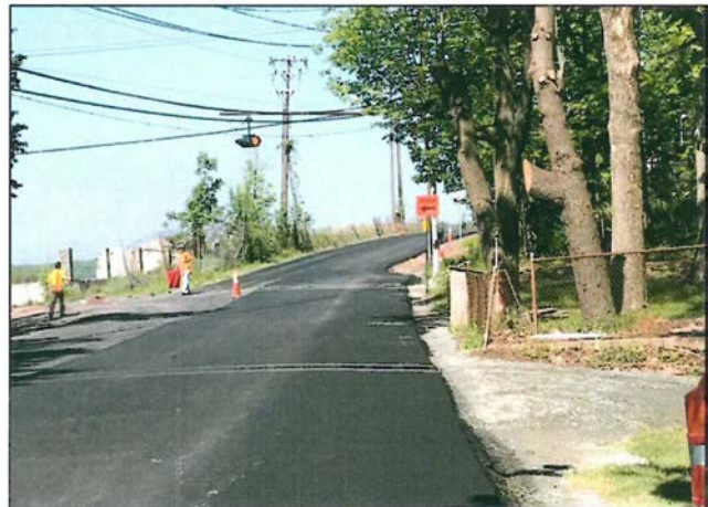
CR 109-Finished Top Coat
