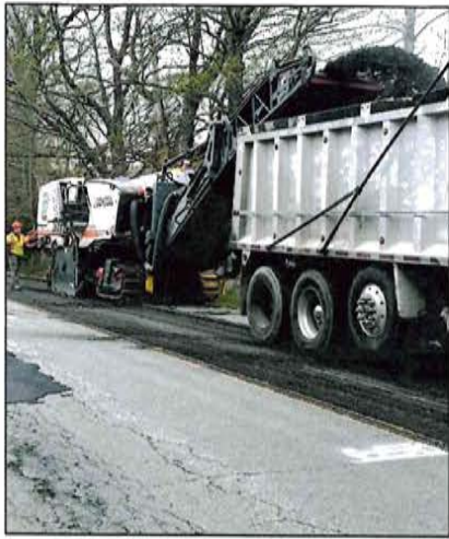
County Road 58 Milling Repairs
