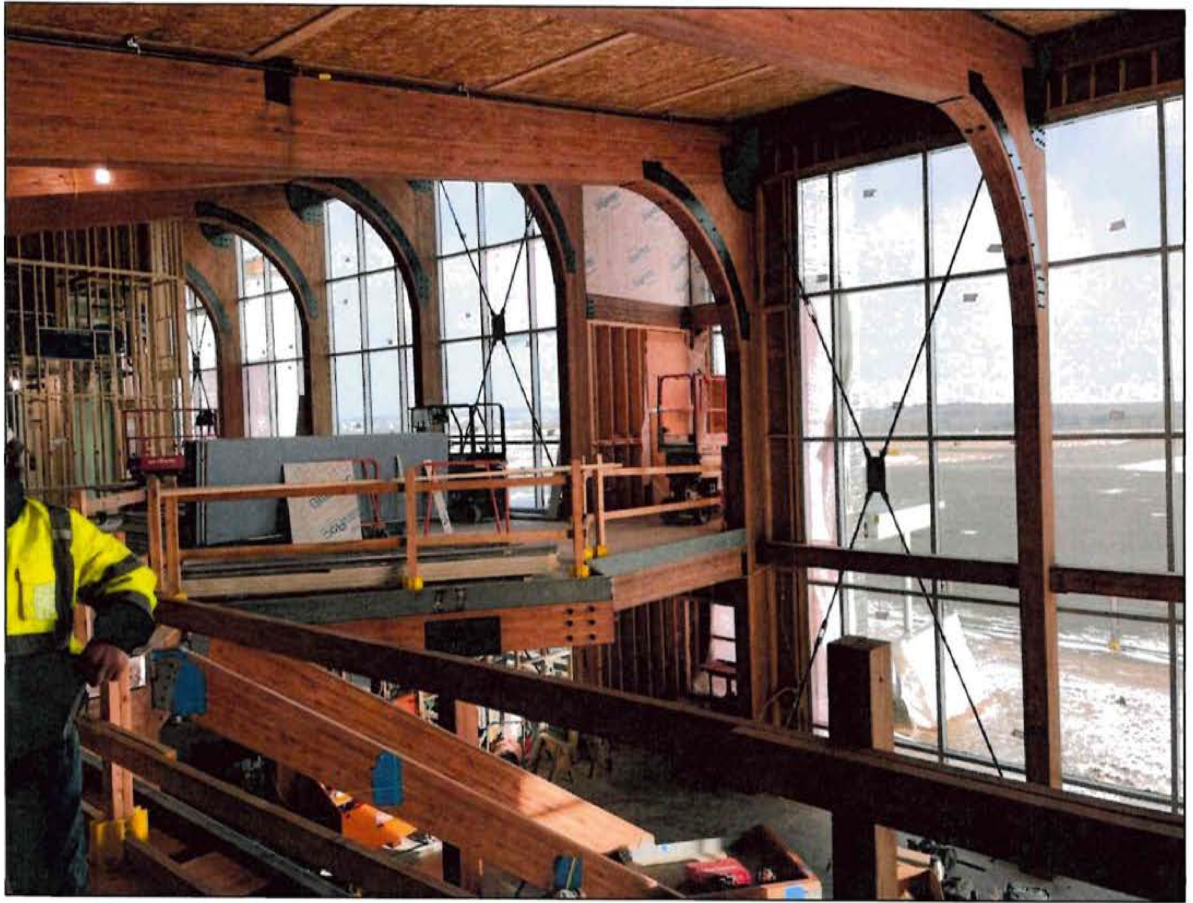
Airport Terminal Second Floor Office Balcony to Dining Space View
