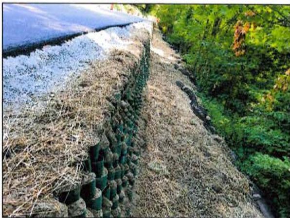
County Road 94 Embankment Repair - GRSS Geo-Cell Retaining Wall
