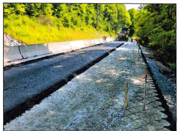
County Road 94 Embankment Repair - GRSS Geo-Cell Retaining Wall
