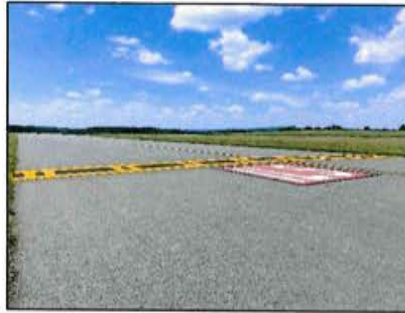
Taxiway A – Line Painting (ILS Hold Marking)
