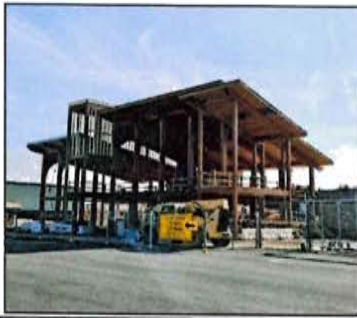
Terminal Building Construction Project
