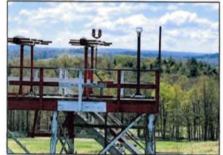
DME Installation Project
