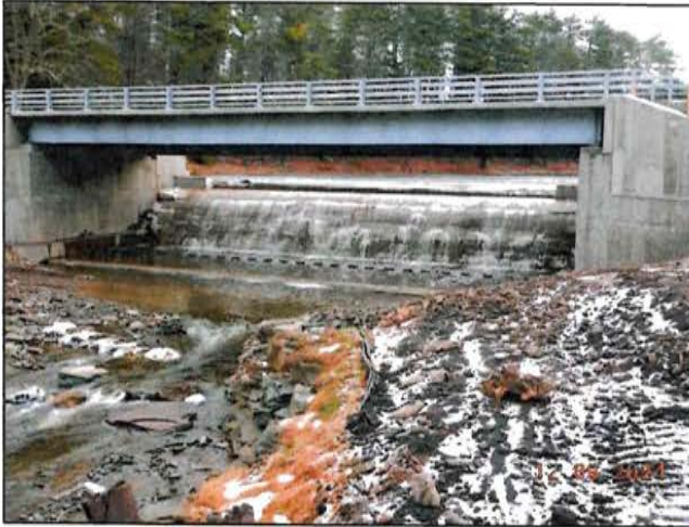
New Bridge 77 Shown on County Road 22/Eldred-Yulan Road in the town of Highland with a new Dam Spillway. Typical Example of Successful Procurement of 95% funding and Contract Administration.
