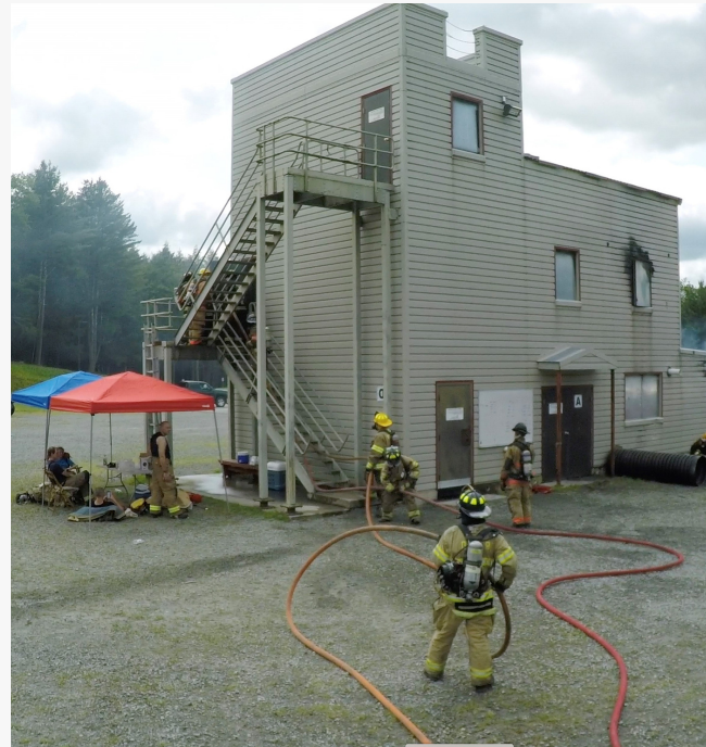
Firefighters practicing on a reusable simulator at our Fire Training Facility in White Lake
