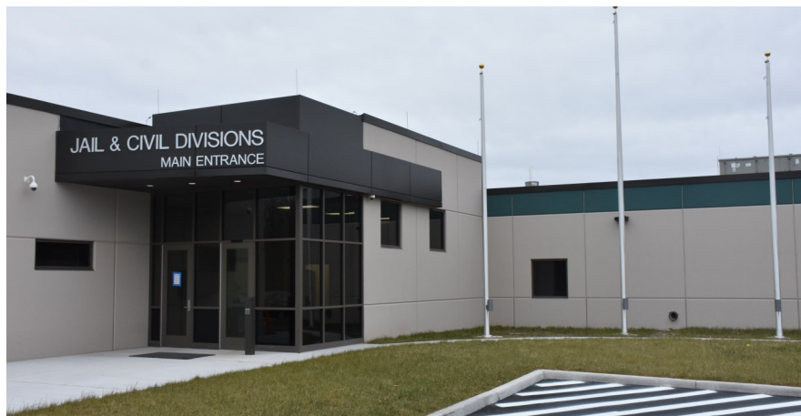
The lettering and lighting are in place for not only the new Sullivan County Jail but the Sheriff's Office relocated headquarters (including the Civil and Patrol divisions).
