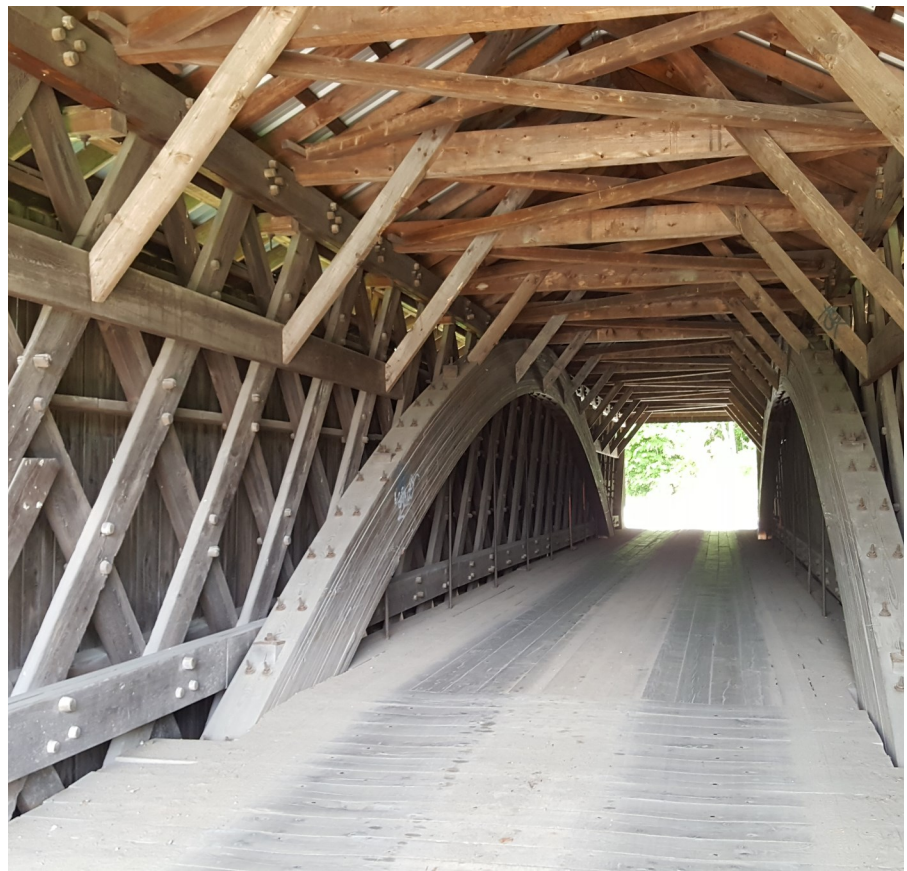
The Livingston Manor Covered Bridge has spanned the Willowemoc since 1860.
