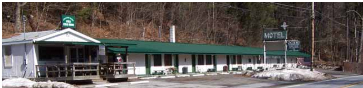
One of the several businesses located in Pond Eddy
