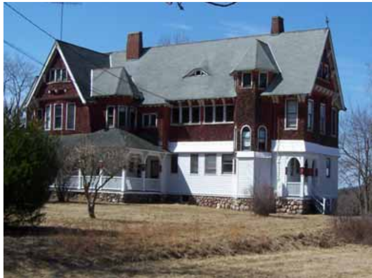
Historic Mansion, now a summer camp, located on Route 41, the High Road
