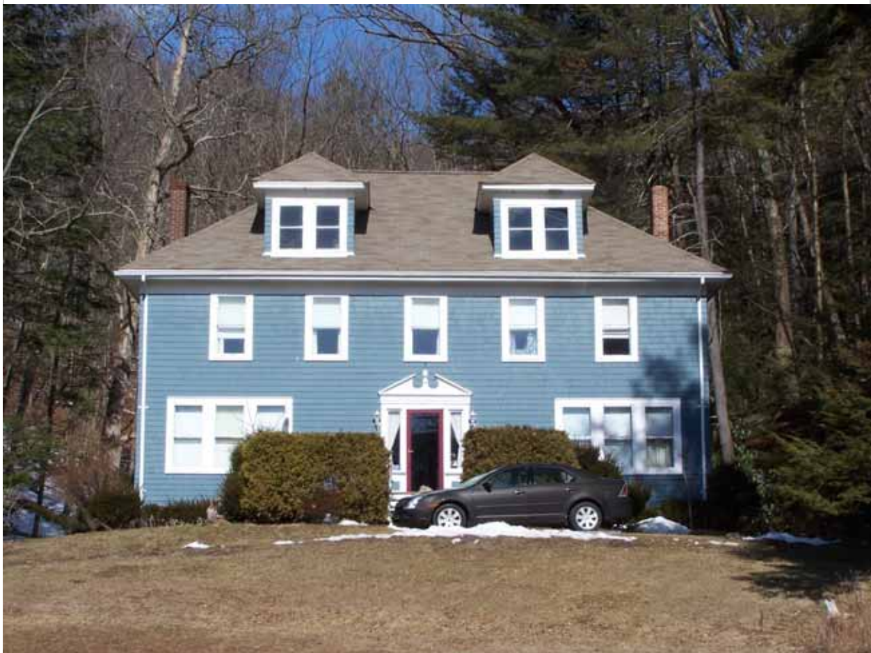
House tucked in below the ridgeline with a view of the Delaware River
