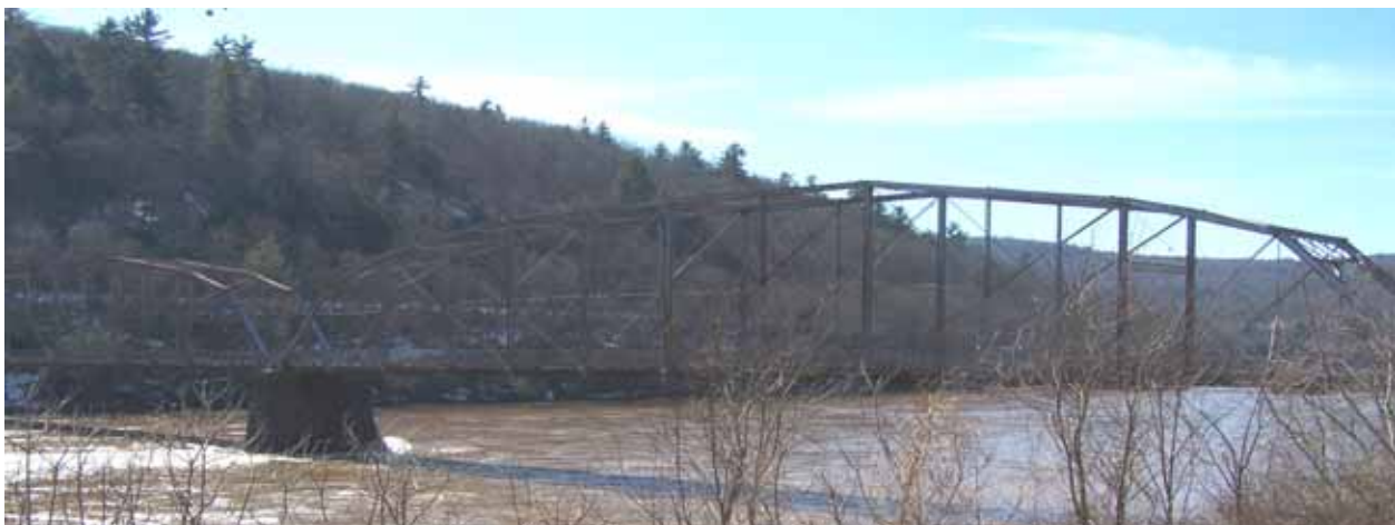
Pond Eddy Bridge
