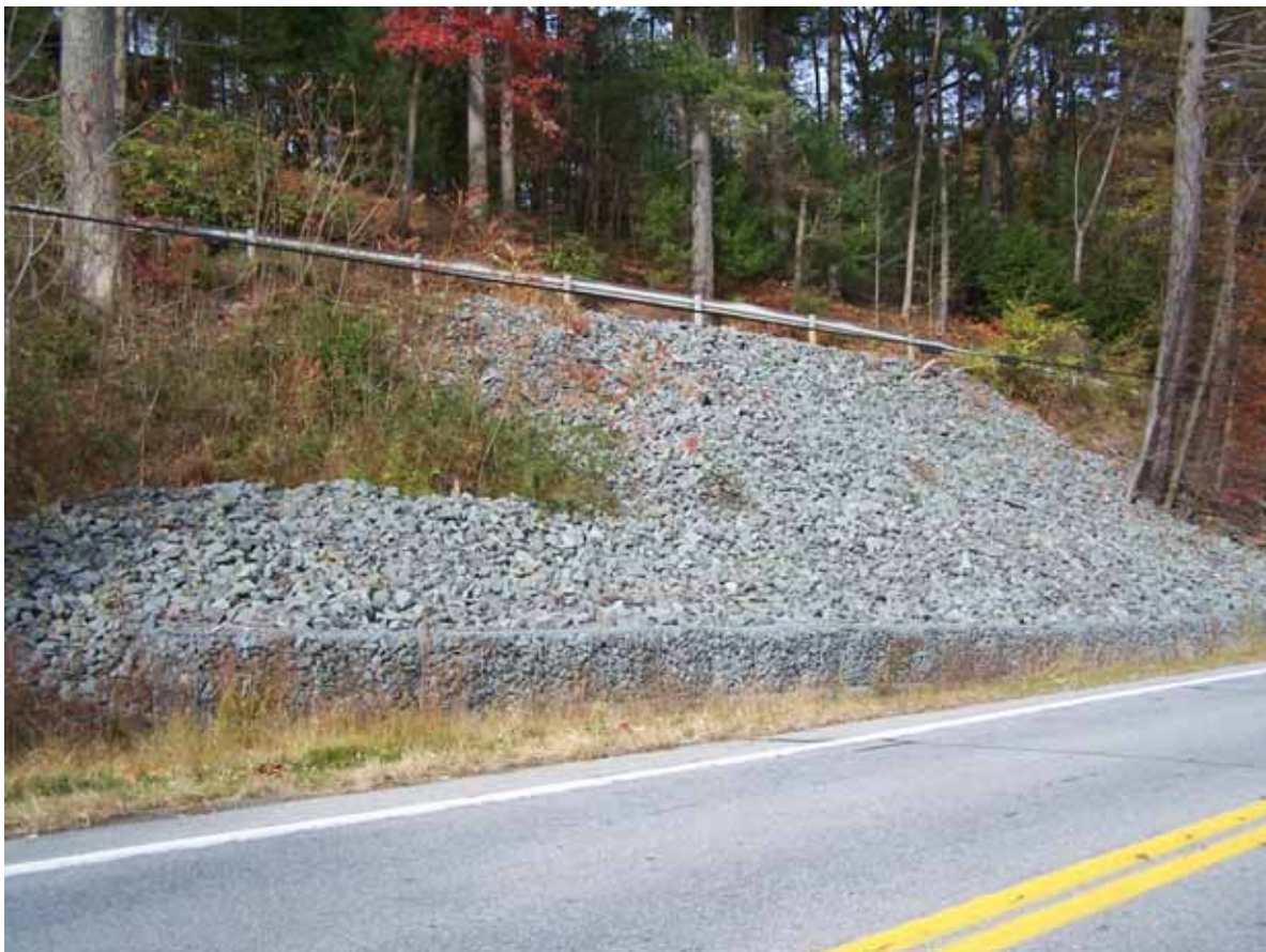
Erosion mitigation along Route 97 in Lumberland
