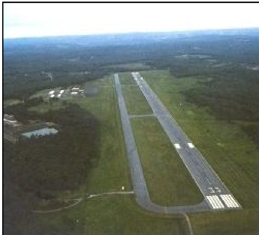
Figure 2.13 – Aerial Image of the Sullivan County International Airport (Sullivan County Division of Public Works, 2010)
