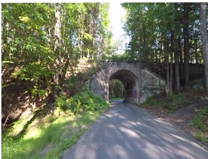
Bridge at Red Hill Road
