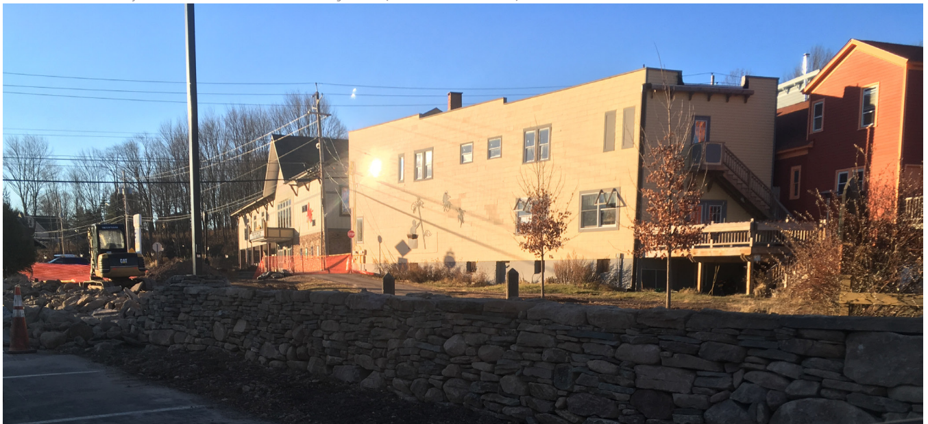
Construction adjacent to the trail in Hurleyville (November 2017)
