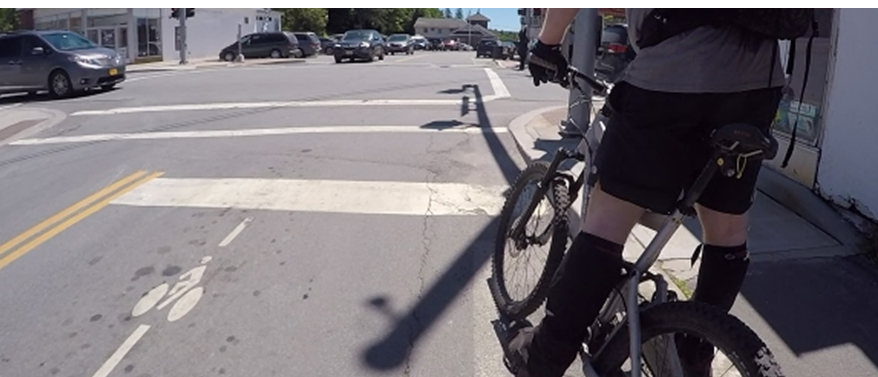
Undersized pavement markings in South Fallsburg
