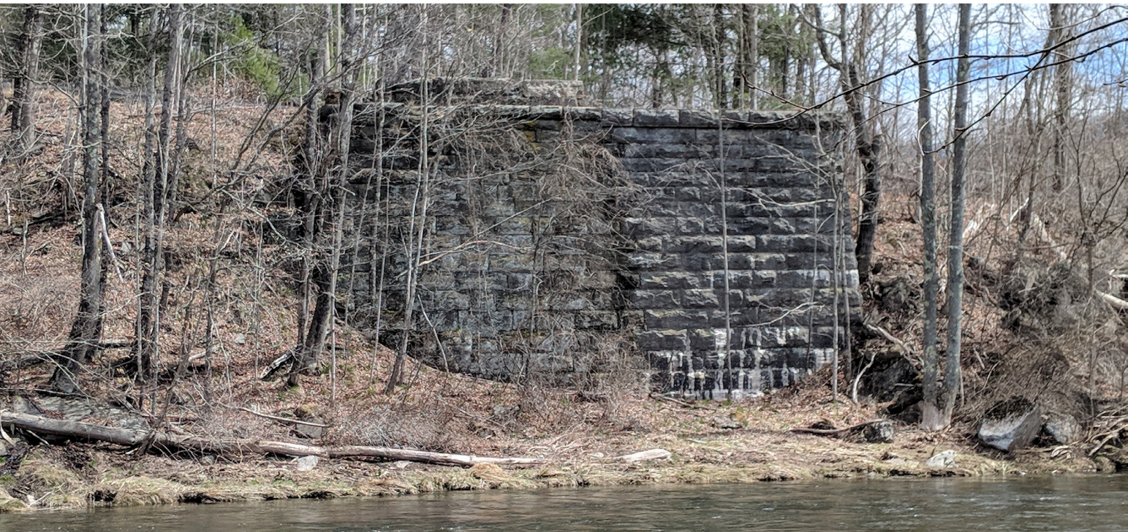
Bridge Abutment at the Neversink River
