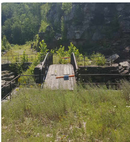
Existing bridge at Tomsco Falls
