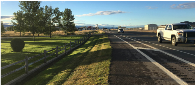
A wide paved surface, paired with a buffer area provides a more comfortable experience for bicyclists travelling on this shoulder.
