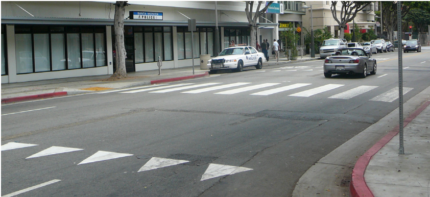
Yield line clearly indicates expected behavior at this mid block crossing.
