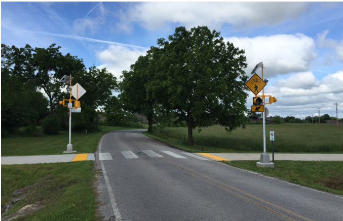
This path crossing includes many enhancements to slow traffic and promote yielding.
