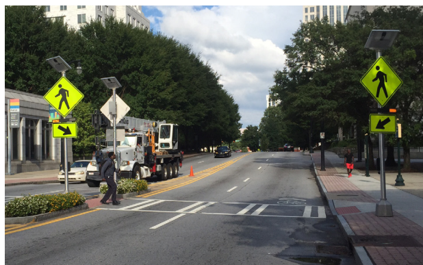
On multilane streets, multiple beacon installations are critical for awareness by motorists in all approach lanes.
