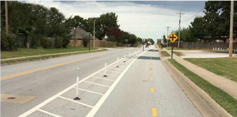
Some segments of the Razorback Greenway Trail operate in the roadway, with minor physical separation between the roadway and the trail.
