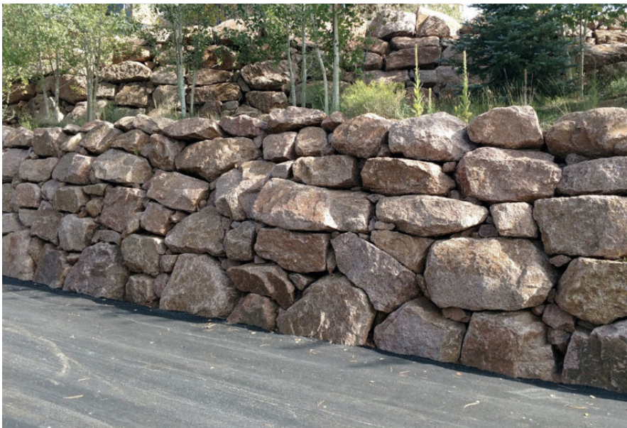
Boulder Retaining Wall at Woodland Park (Source: Bantly's Landscape & Design, via http://www.bantlyslandscape.com/gallery/ )
