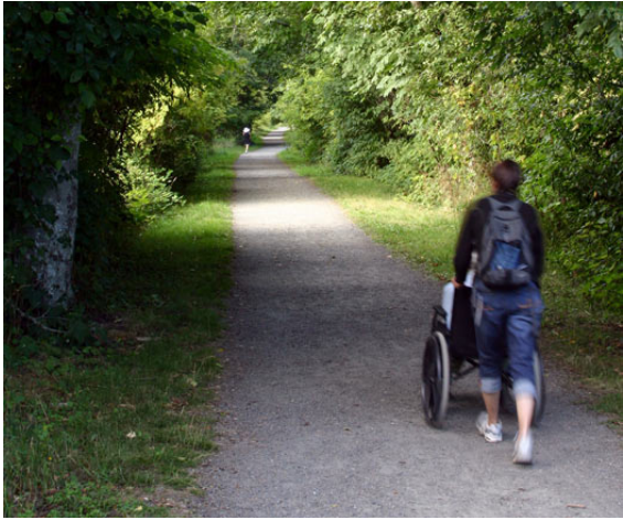
Smooth crusher fines can be a good surface material for natural surface trails for all user types (Source: National Trails Training Partnership)
