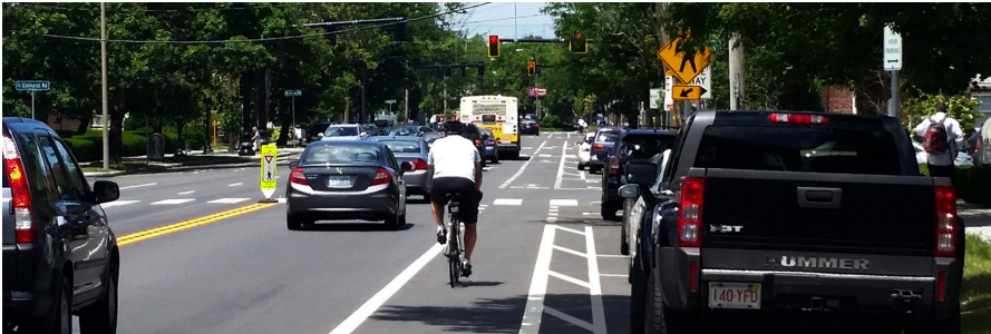
A 2 foot buffer between the bike lane and the parking lane increases the distance from the door zone of parked cars.
