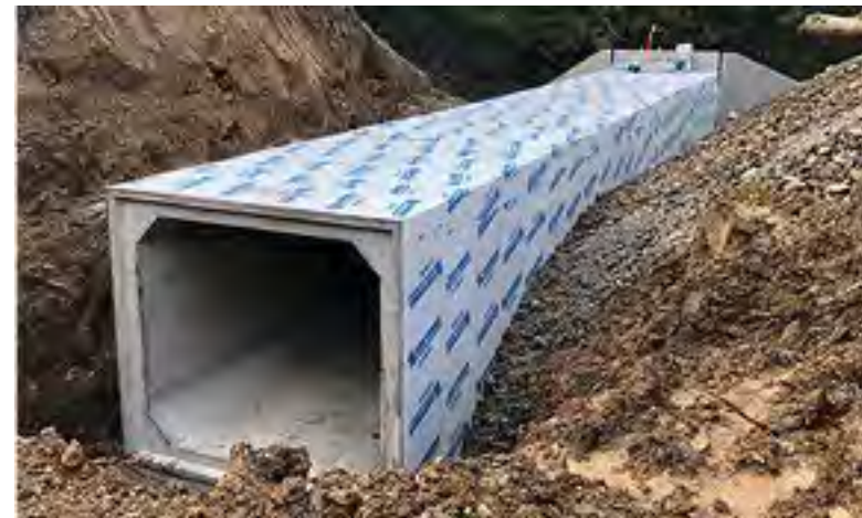
Example of four-sided box culvert recently installed and ready for backfill
