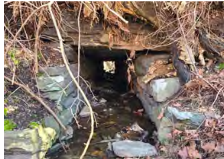
Original O&W stone culvert
