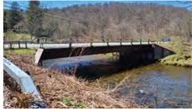
Dahlia Road bridge over the Little Beaver Kill
