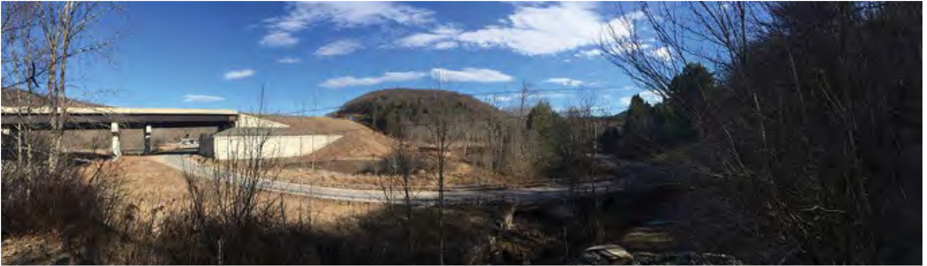
View looking from the original O&W bridge abutment above Fox Mountain Road
