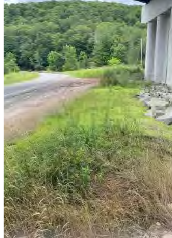
Existing bridge piers of the Route 17 WB overpass
