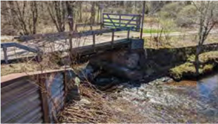
Looking north on Dahlia Road where overhead utility wires would be in direct conflict with the proposed bridge over Dahlia Road
