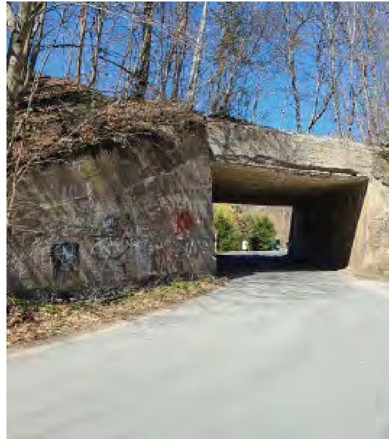
Existing bridge over Old Liberty Road
