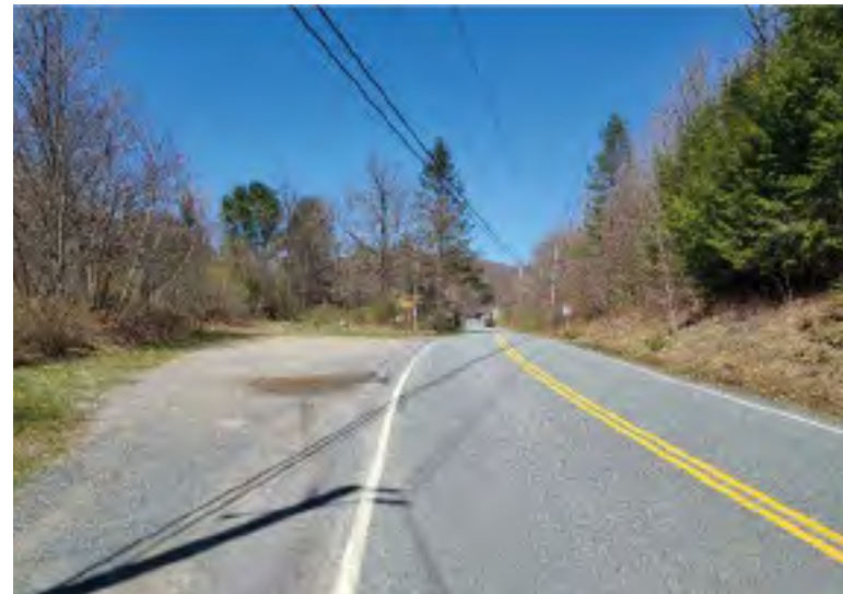
Looking north on Dahlia Road where overhead utility wires would be in direct conflict with the proposed bridge over Dahlia Road
